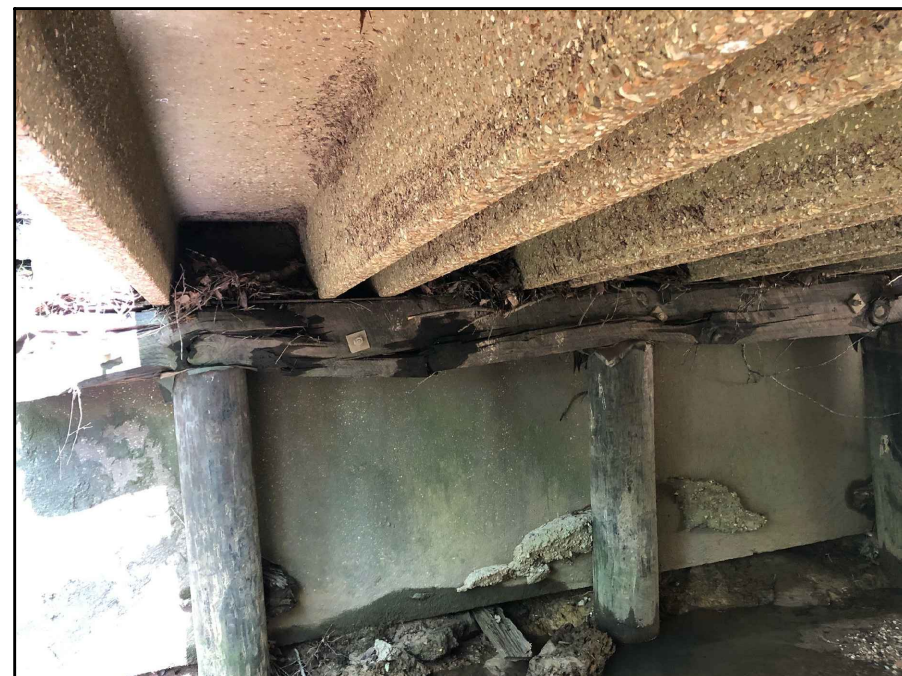
SECTION OF CAP TO BE REPLACED
